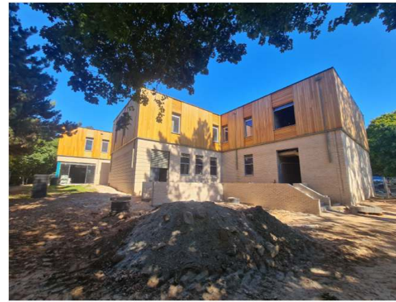
Dartmouth Health Hub: image extracted from August 2022 Contractor Report
